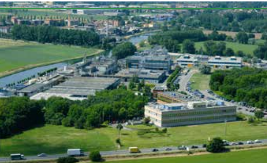
Indena's Settala production plant. Photo ©2021 Indena
