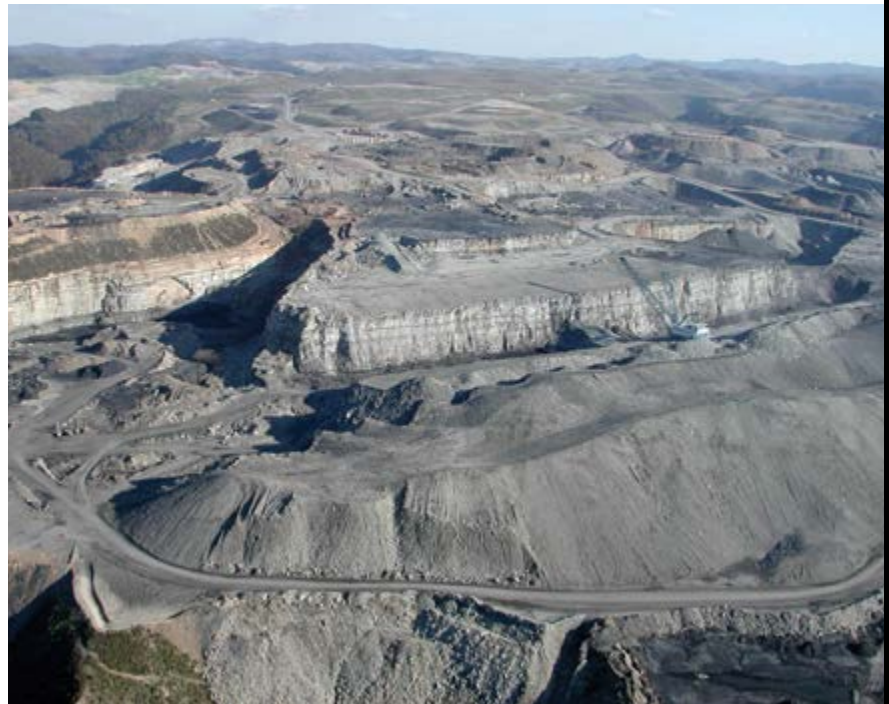
Below: Figure 3. View of Kayford Mountain site, West Virginia, on October 19, 2003. This is becoming a familiar scene in Appalachian coal country with over 380,000 acres of rugged mountains being altered into level, grassy plateaus by mountain top removal operations. Photo © Vivian Stockmen www.ohvec.org .
